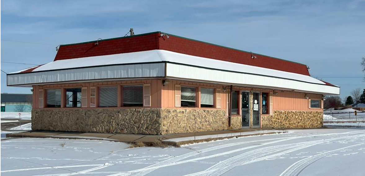
Photo 27 – Photo of the front of the building
