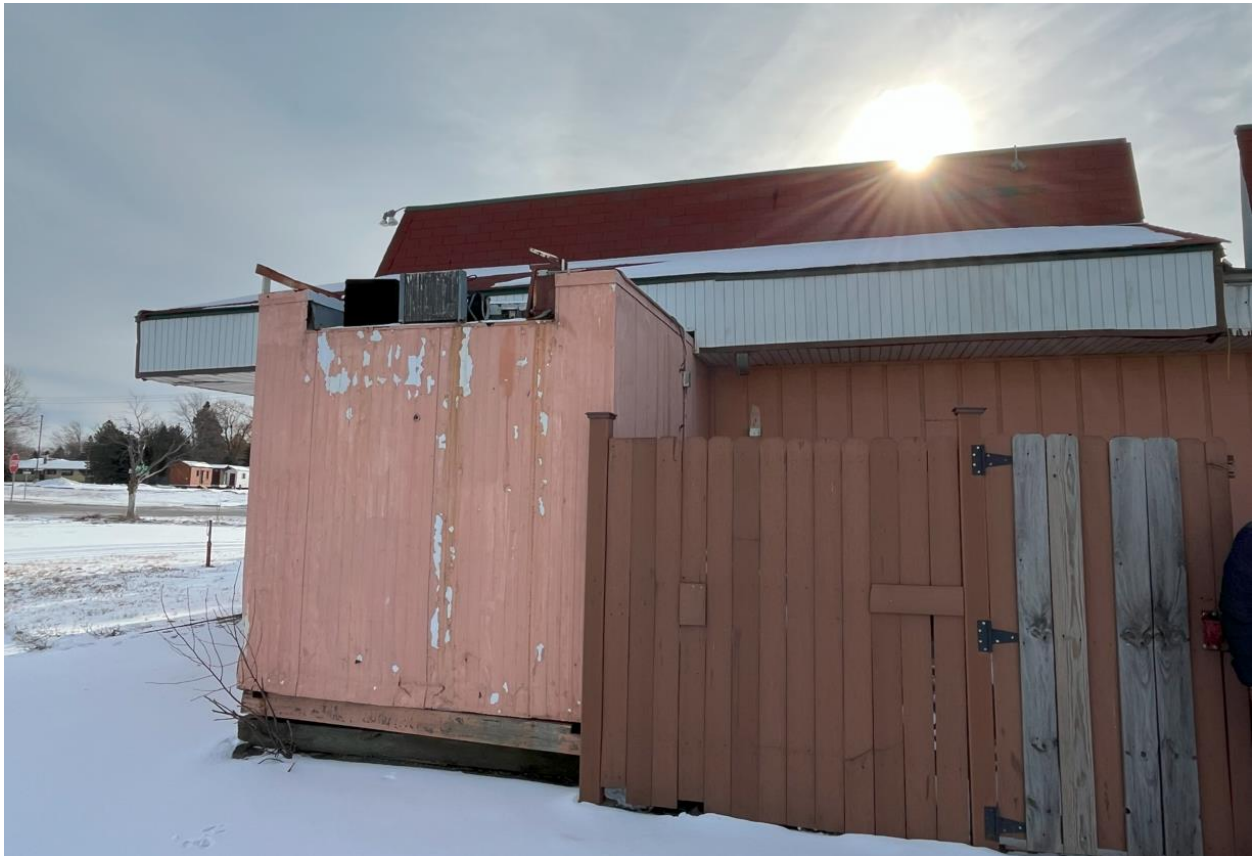
Photo 32 – Cooler addition at the back of the building
