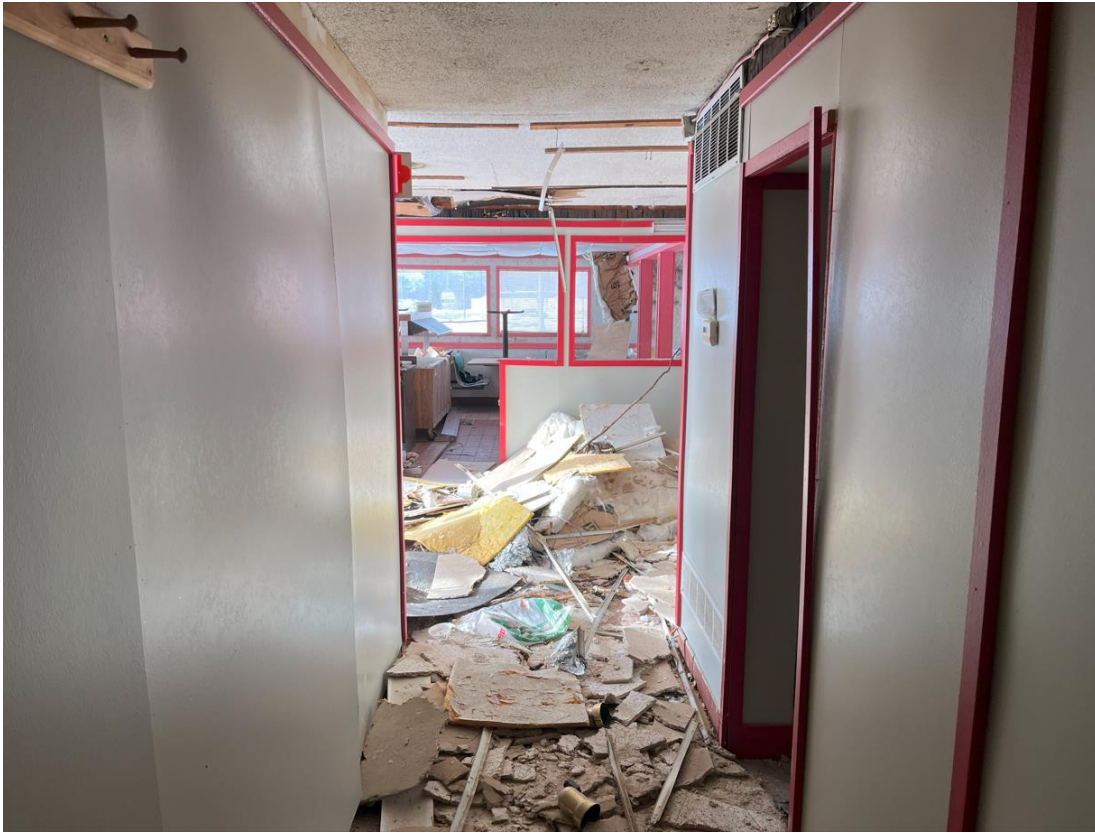
Photo 12 -Looking from the kitchen to the dining room area
