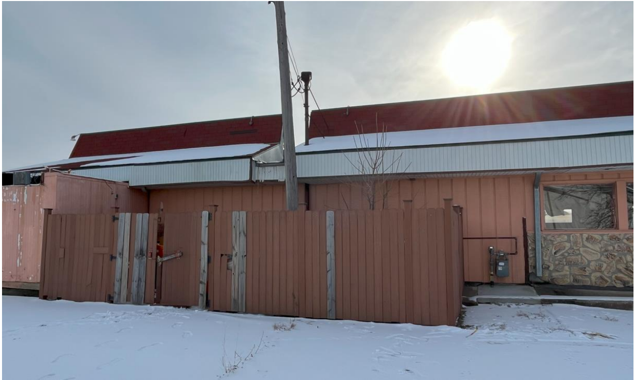
Photo 31 – Back of the building
