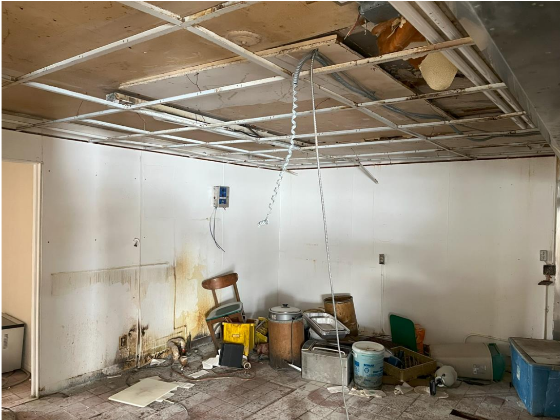
Photo 15 – The sinks and counters have been removed from the kitchen
