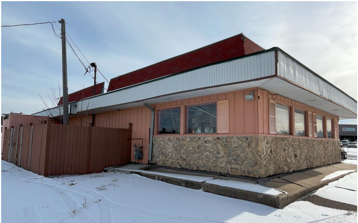
Photo 30 – Back of the building
