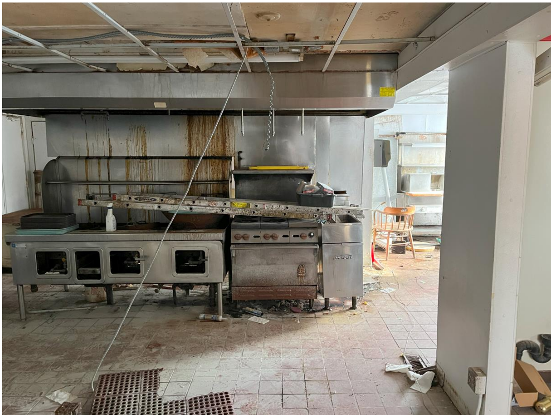
Photo 16 – Photo of the kitchen showing condition of the hood and cooking line
